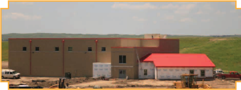
OLC's new Lakota demonstration school in its construction phase
